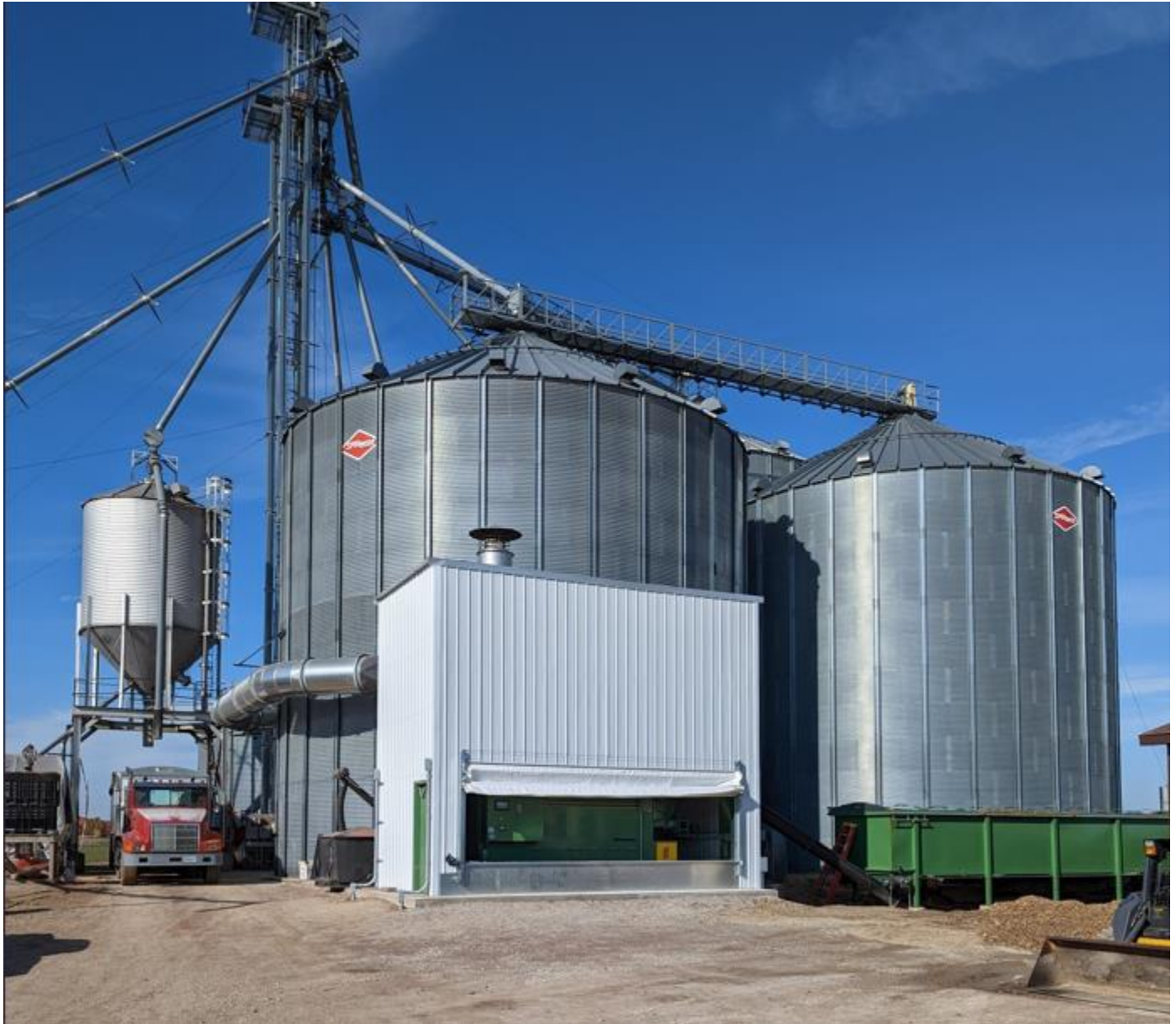
GRAIN DRYER & INFEEED HOPPER SYSTEM
